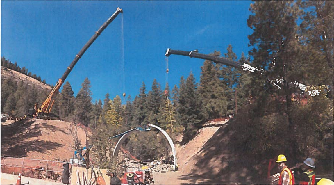
(WSDOT - State Route 12 – M.P. 166 / Wildcat Creek Bridge Replacement Project)
